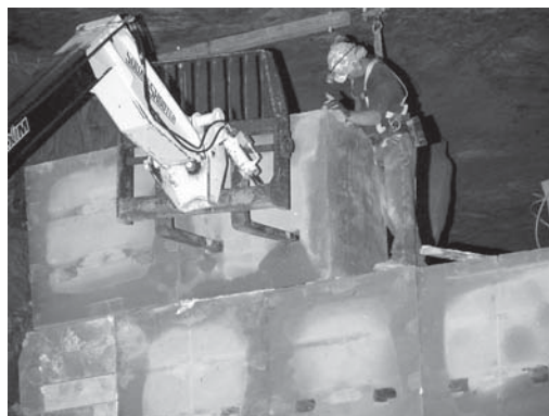
Figure 2. Setting blocks for construction of a Super Stopping using extended reach fork lift and precast lifting holes.
