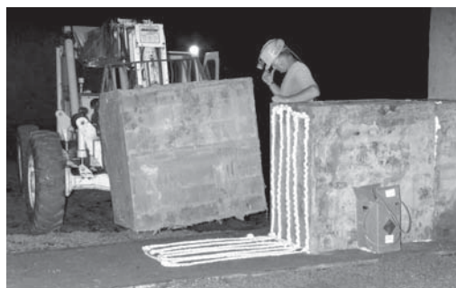
Figure 3. Placing Super Stopping block in place after applying adhesive.
