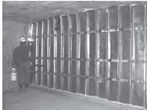
Figure 3. Nearly completed Kennedy steel stopping showing the back side of the panels attached to the horizontal steel angle bars.
