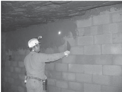
Figure 2. Miner applying sealant to concrete block stopping.
