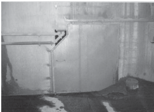
Figure 3b. Seal installed where connecting tunnel accesses main structure in basement of facility.
