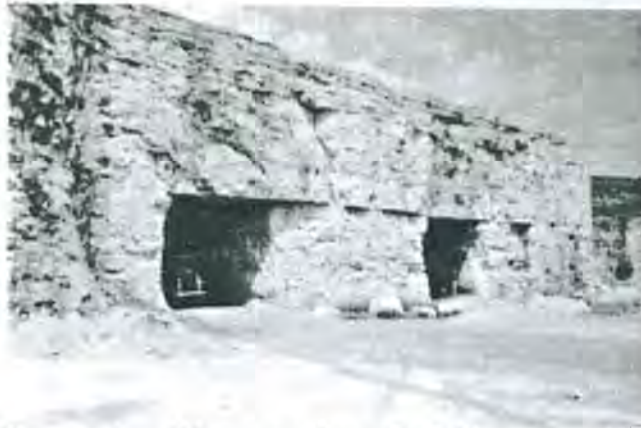
Figure 4. Smooth roof line produced by a persistent bedding plane lamination within the roof rock beam
