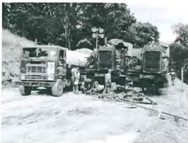
Figure 3 Inert Gas Injection at Loveridge Mine
