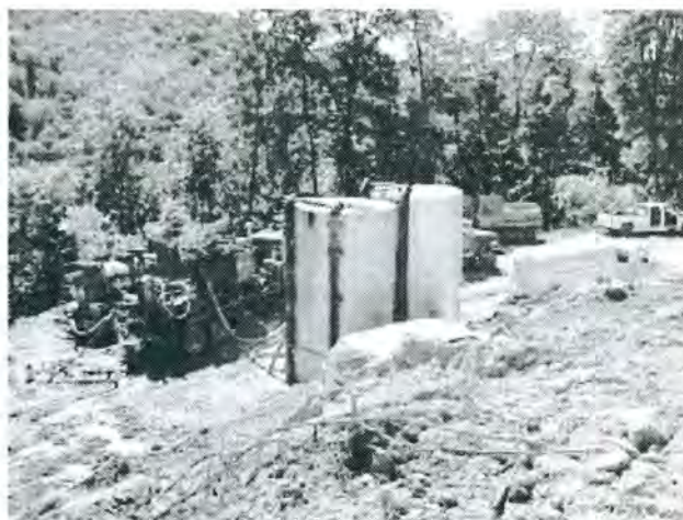
Figure 4 Surface Seal Construction Site
