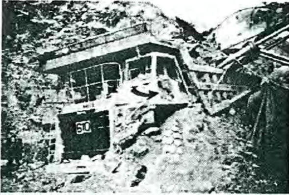
Figure 2. Consequences of unexpected slope failures.
