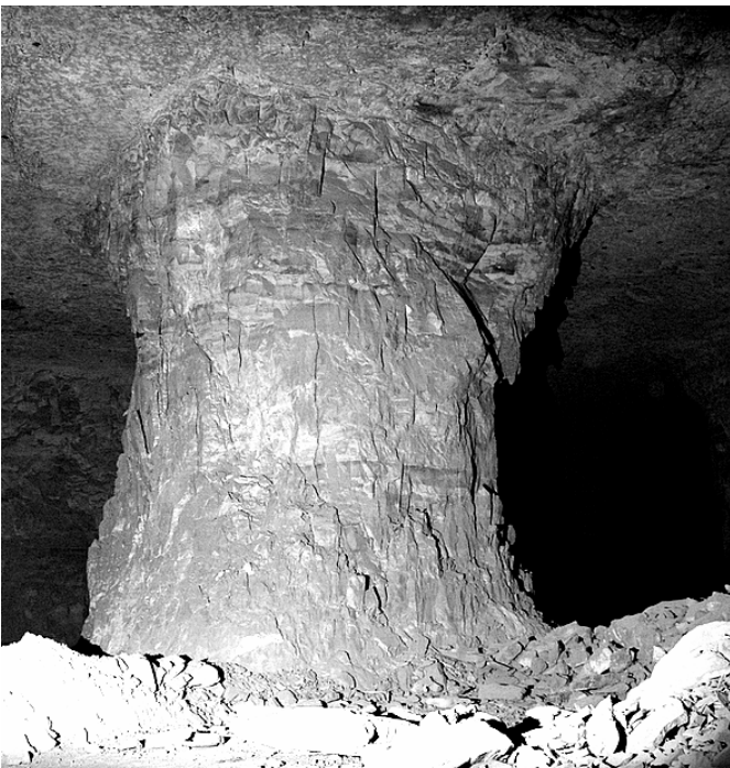
Figure 9. A pillar with a width to height ratio of 0.77 showing the effect of brittle failure and spalling. Open vertical fractures/joints are visible in the pillar.
