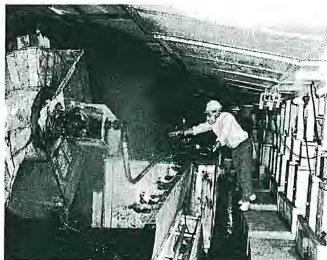
FIG 9 - Testing in full-scale longwall dust gallery.
