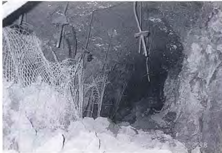
Figure 7. Rock burst damage in the 5750-05 stope. Note that both ribs and the overhead sandfill were damaged.
