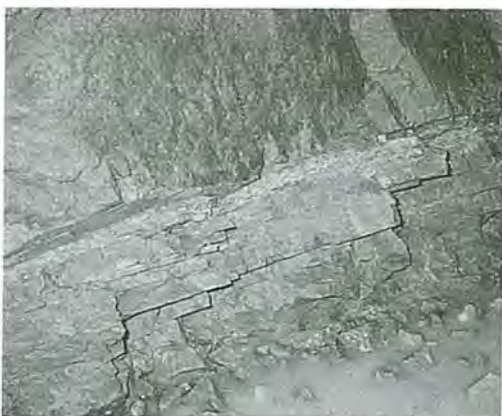
Figure 2. Soft, white gouge on slip plane in argillite interbed in hanging wall rib.
