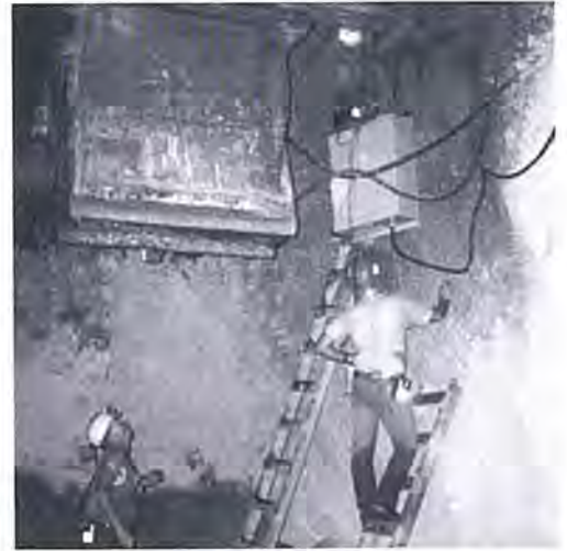
Figure 3. Instrumenting support bolts at truck loadout chute.
