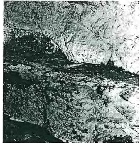
Figure 6. Example of differential movement along parting in coal rib.
