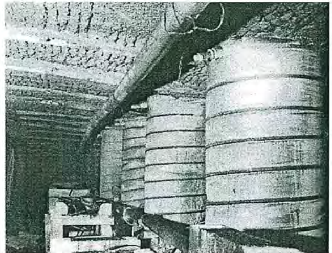
Figure 11b. Inby area supported by pumpable crib.
