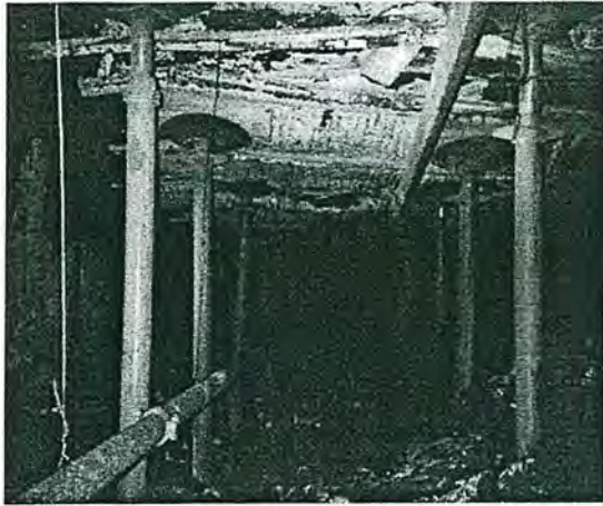
Figure 13b. Inby area supported by ACS supports.
