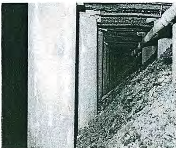
Figure 14b. Inby area supported by the Can Support.
