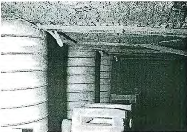
Figure 11a. Outby area supported with pumpable crib.
