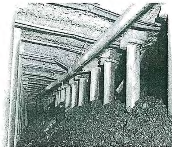
Figure 12b. Inby area supported by Propsetter support.
