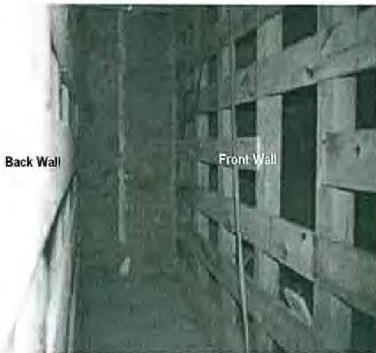
Figure 4.: Photo of inside of Mine Seal No. 1 showing the wooden form.
