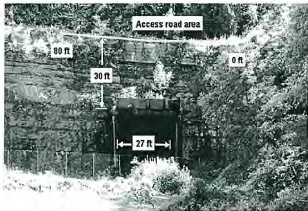
Figure 7. Photo of Portal No. 4 at the Lake Lynn Experimental Mine (Site 2). Note relative position of GPR survey line is shown at the top of highwall.
