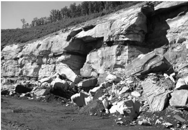
Figure 13. Highwall collapse in multiple seam mining area
