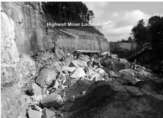
Figure 3 – Highwall collapse resulting in fatality.
