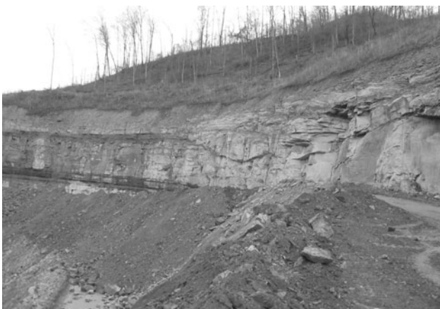
Figure 14. Highwall collapse in multiple seam mining area.
