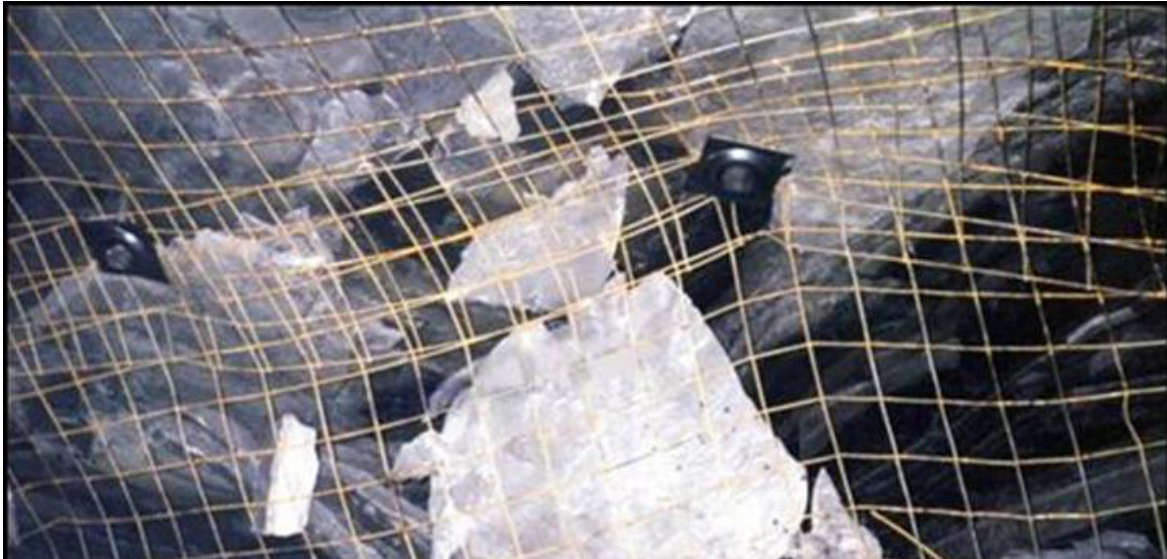
Figure 4. Roof screen can hold up large pieces of broken roof.
