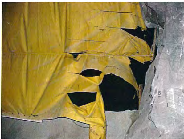
Figure 7. Typical repetitive flapping damage caused by static pressure across stopping (not blast damage)
