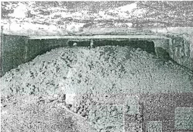
Figure 9. View of bulk fill placement for seal No. 2.
