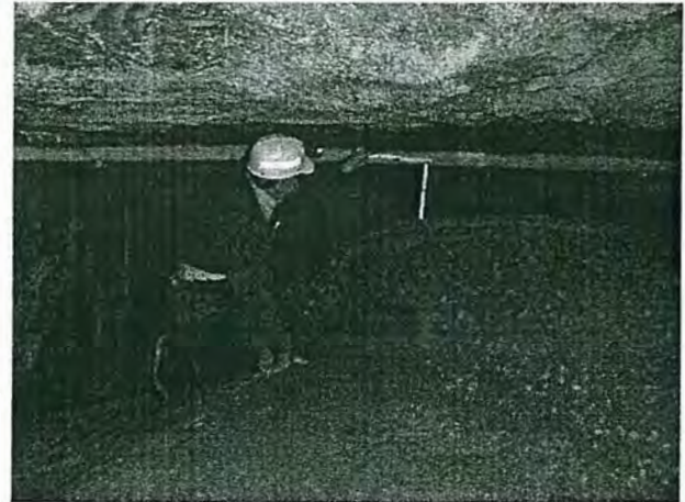
Figure 5. Underground view of bulk fill material for seal No. 1.
