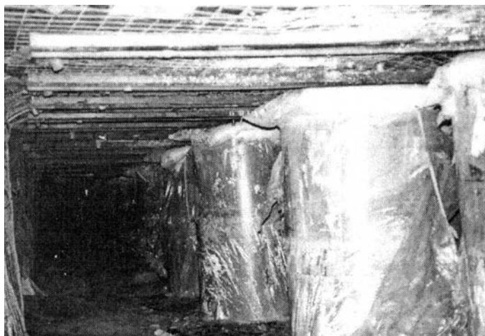
Figure 6. Photograph of completed cribs, roof supports, and instrumentation.
