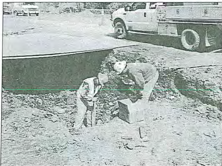
Figure 4 - Steel plates cover the open trench area.
