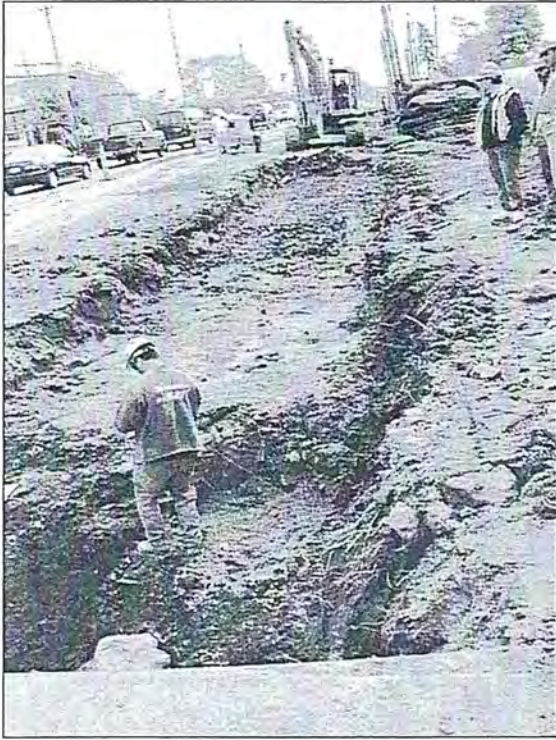
Figure 5 - Overburden is removed from the rock.
