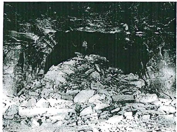
Figure 3. Massive roof fall measuring 45 ft wide by 20 to 30 ft high and extending for approximately 200 hundred feet.
