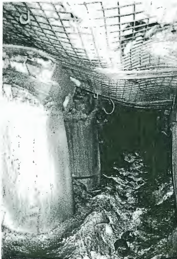
Figure 4. Compressional failures of mine roof and floor due to horizontal stress.
