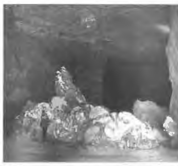
Figure 2 - Large roof fall at underground limestone mine.
