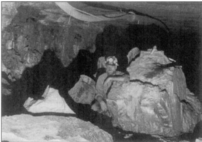
FIGURE 23.4 Large rib failure in a thick coal mine seam (photo by Chase)
