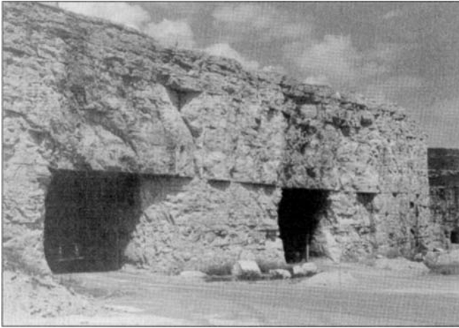
FIGURE 23.11 Smooth roof line produced by a persistent bedding plane lamination within the roof rock beam
