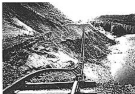
Figure 6. Rail track demolished by a slope failure.
