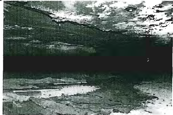
Figure 4. Stress induced cutter roof failure
