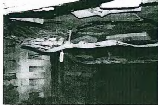
Figure 17. Rear abutment stress damage in L1 entry
