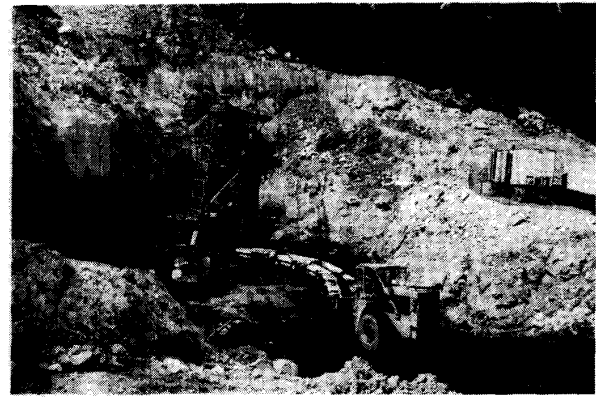
Fig. 8. Teleoperated highwall mining system at production site.
