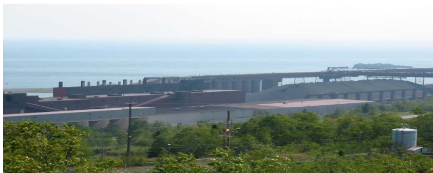
Taconite (iron ore) processing plant in northeast Minnesota along the northern shore of Lake Superior
