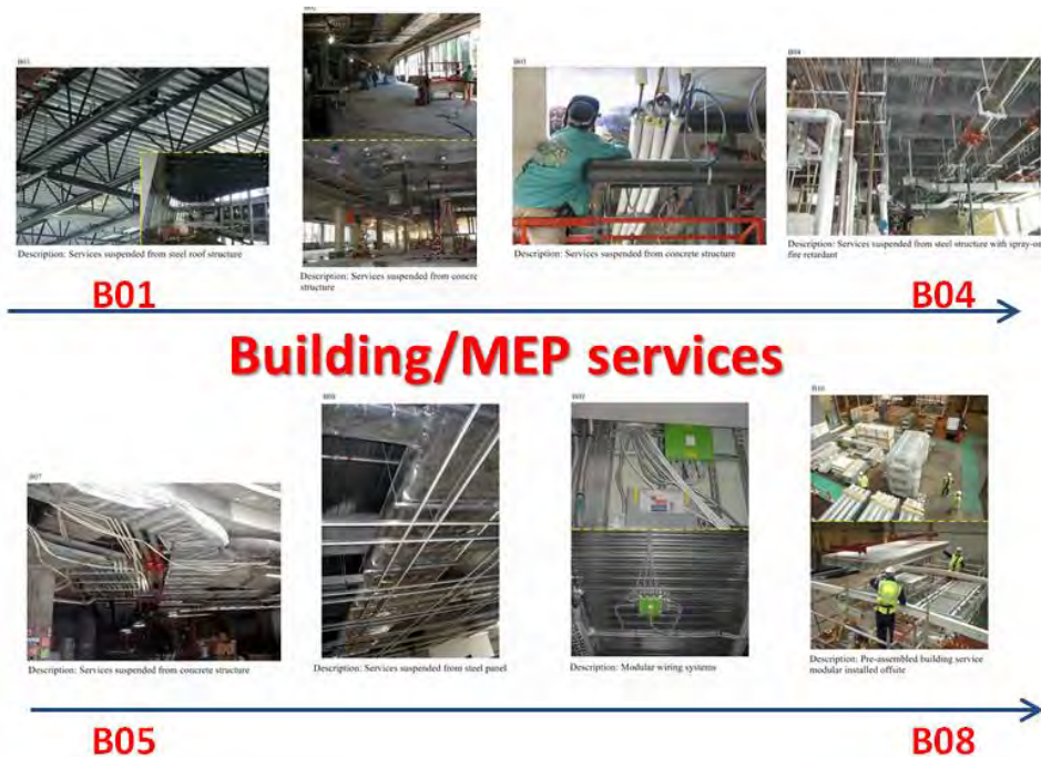
Figure 4. Q-sets photos for façade, roof, structure, and MEP services.
