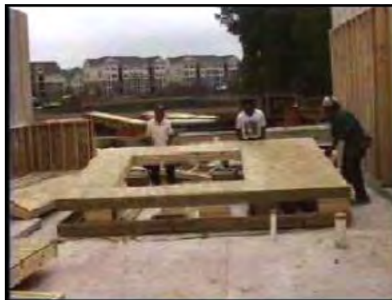
Figure 1.1. Workers lift a sheathed panel from a stack on a pallet.
