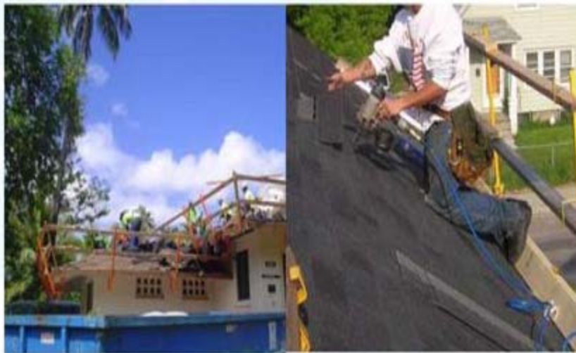
Guardrails in place during re-roofing activities.
