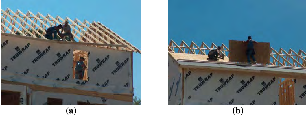
Figure 27: Field Observations of Workers Walking on Individual Wood Elements
