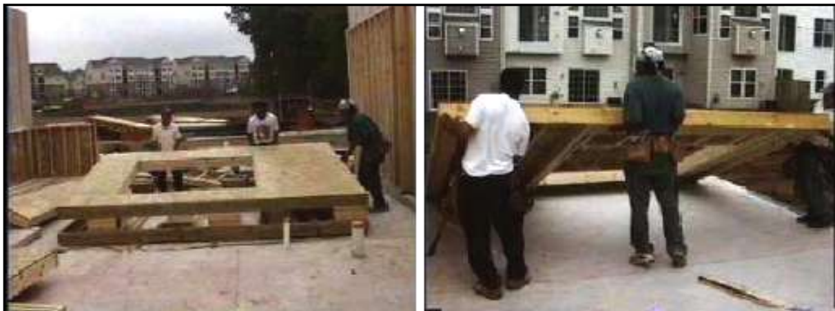
Figure 1.2: Workers lift a sheathed panel from a pallet (left) and into a vertical orientation (right).
