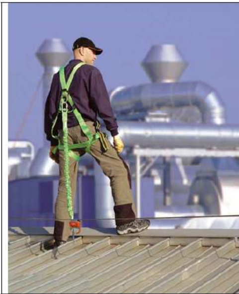
Figure 5. A worker demonstrating the proper fall protection (www.meico.cz)
