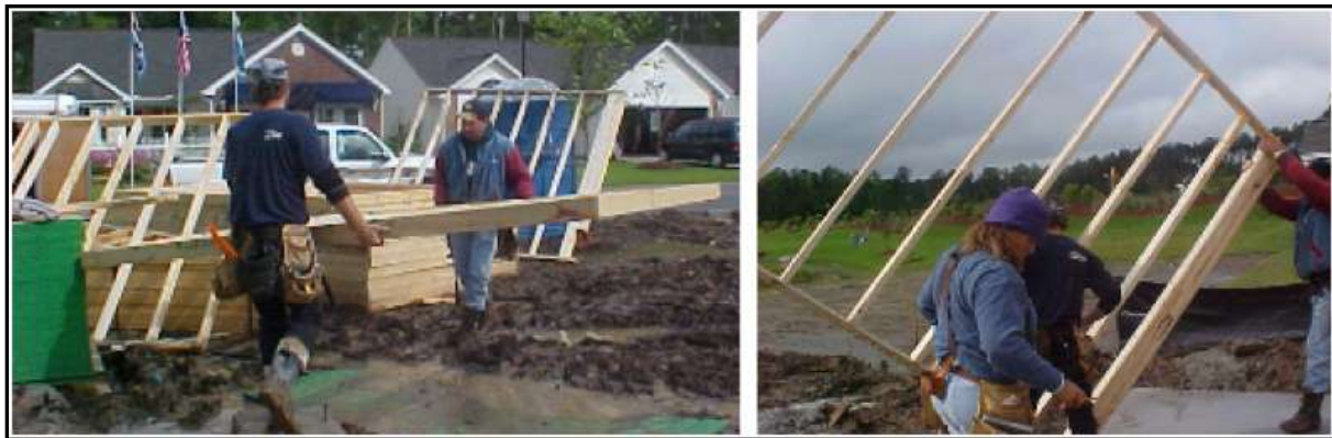
Figure 1.1: Workers remove wall panels from delivery pallet (left) and position panel at installation point (right).
