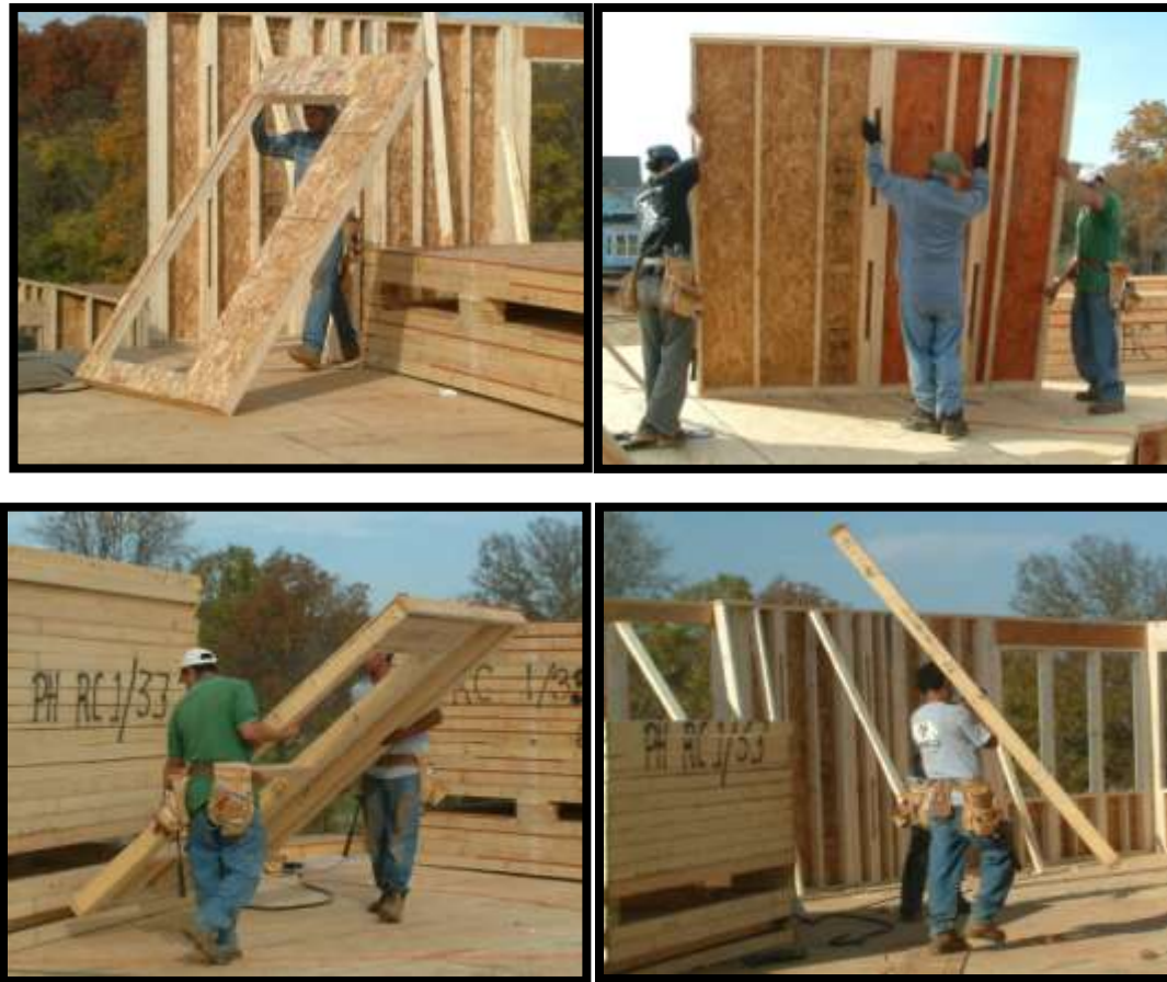
Figure 4.5: Erecting (Above: E1, Below: E2).
