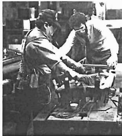
Figure 1-1. Traditional method for moment arm measurement.
