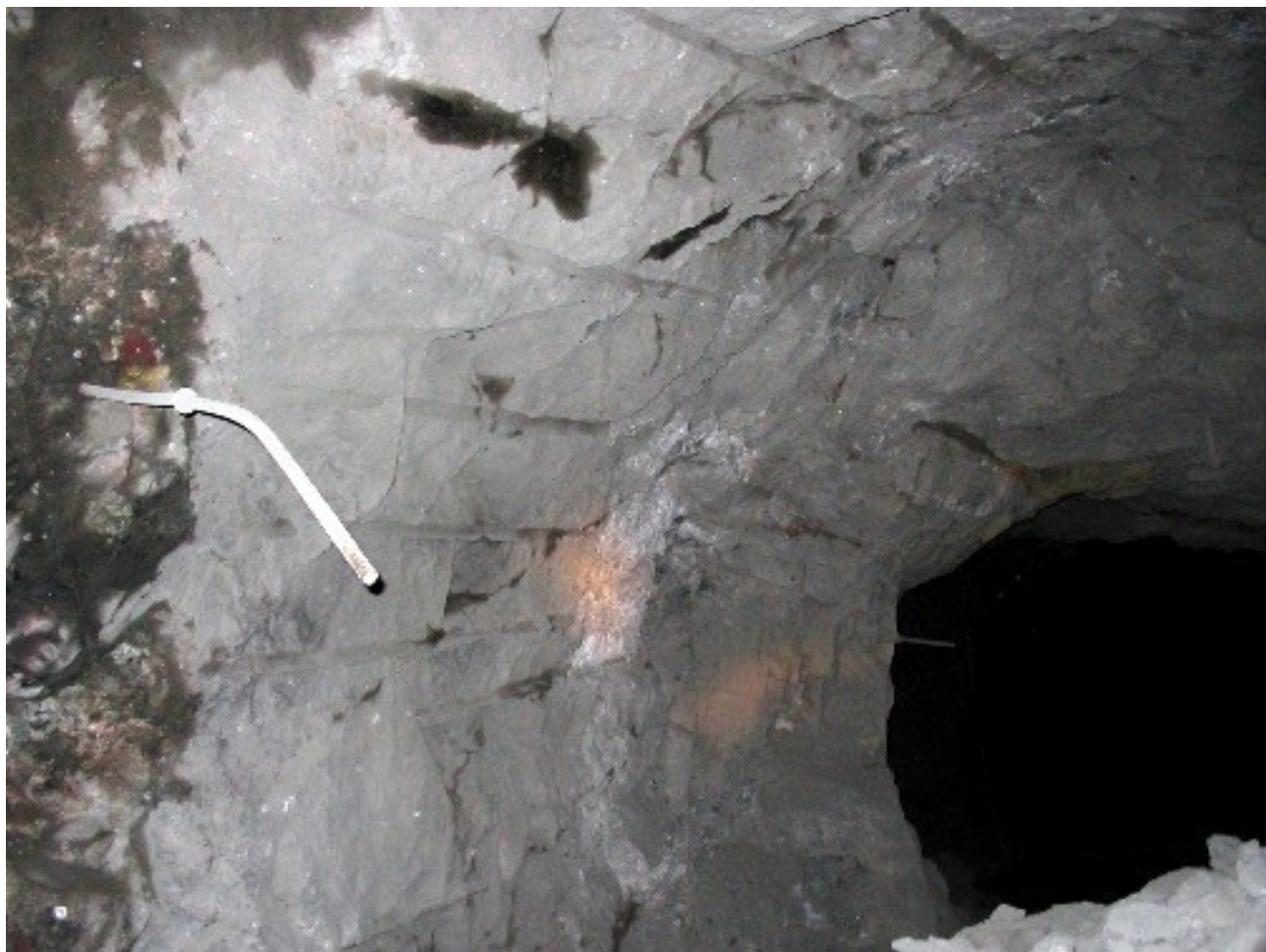
Fig. 11.5. Half-cast drill holes visible after a smoothwall blasting in experiment six.
