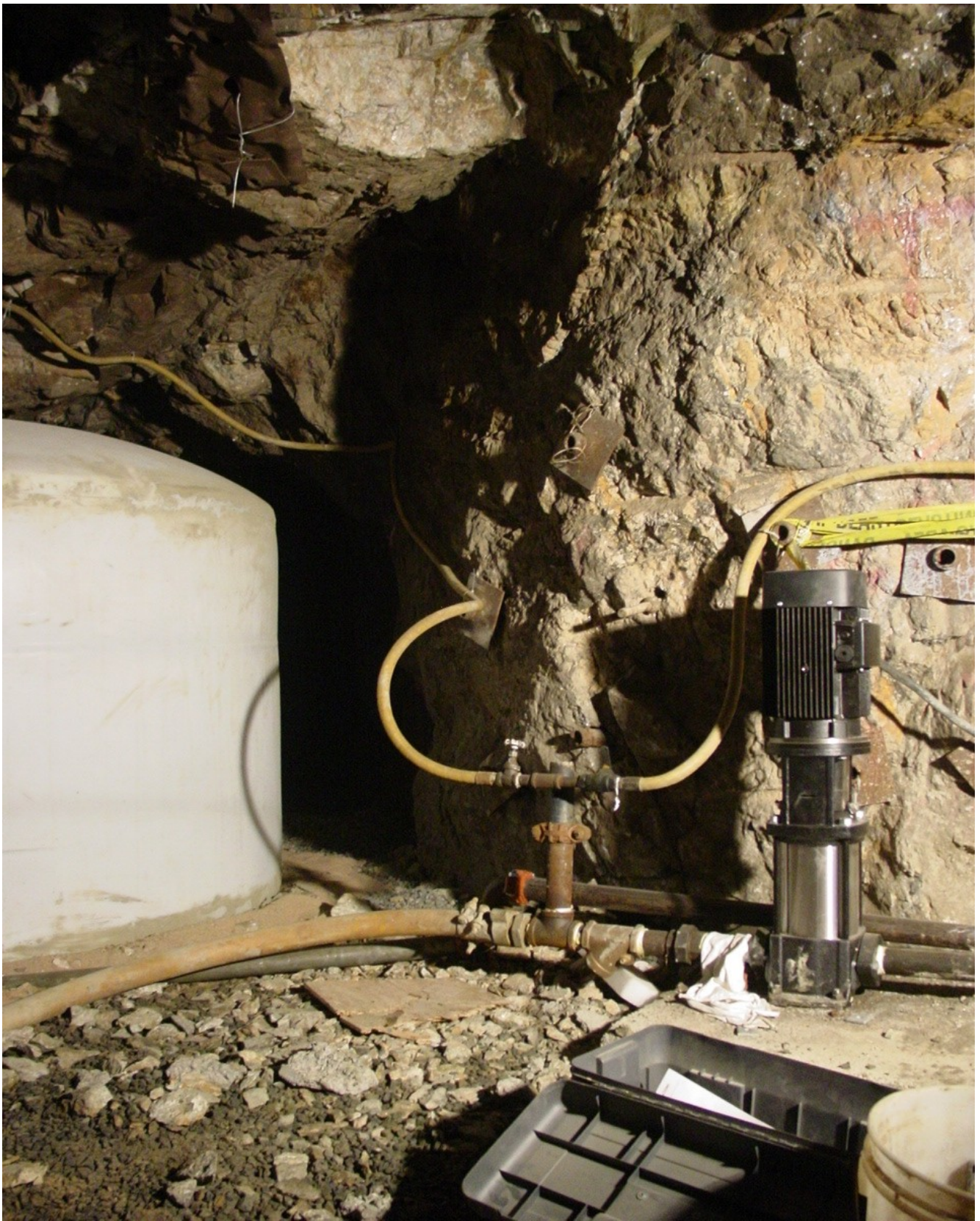
Fig 7.1. Low pressure pump and plastic storage tank that provide water to the high pressure pump.
