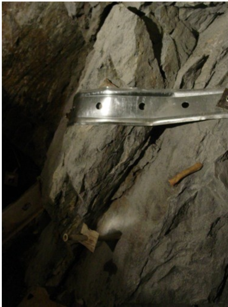
Fig. 10.39 Large slab bound by open discontinuities
