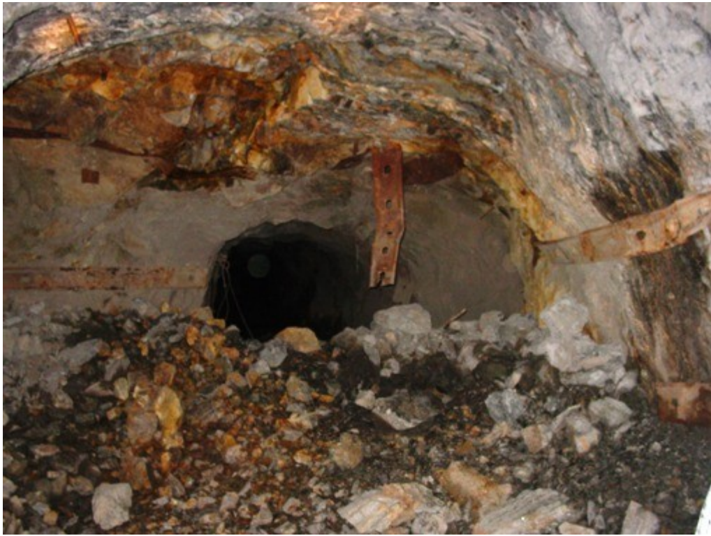
Fig. 10.38 Fractured and weathered weak zone in Experiment #8
