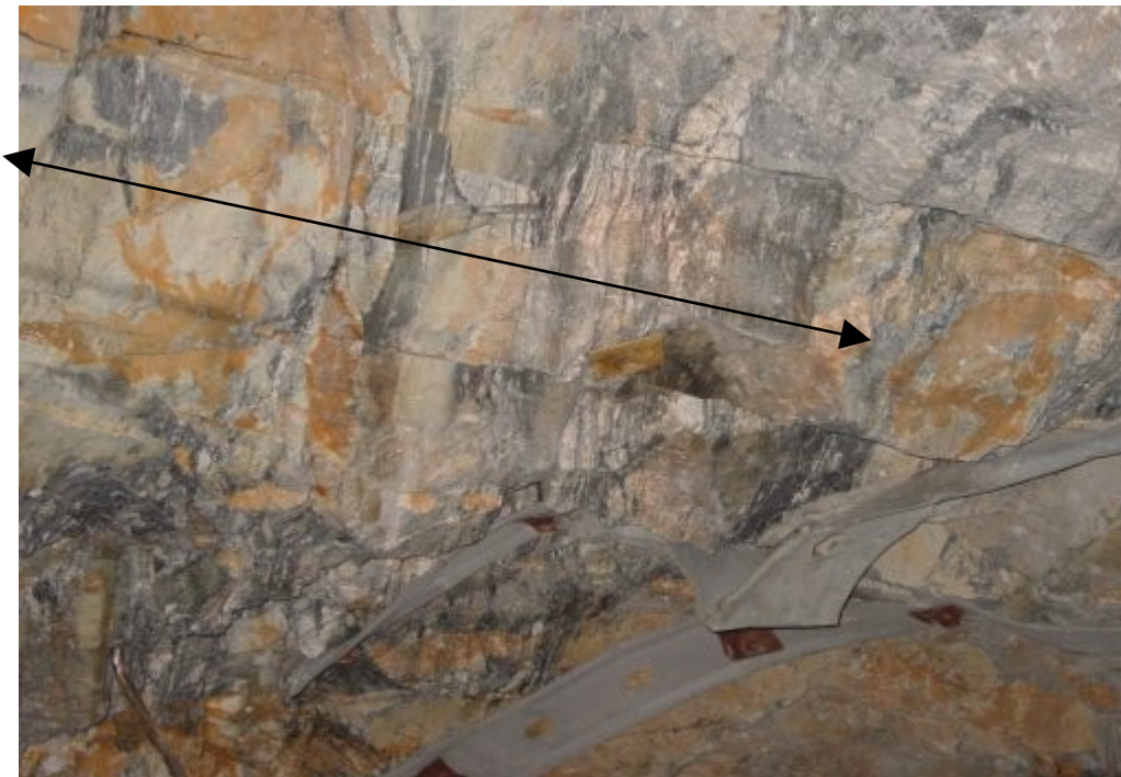
Fig. 10.9 Troubling discontinuities noted before Experiment #2
