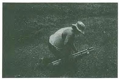
This task involves using a post hole digger. A non-automated post hole digger weighs approximately 40 lbs. A manual post-hole driver weighs approximately 15-20 lbs. A tractor-powered (power take-off) post-hole digger weighs in excess of 500 lbs. The post is manually or automatically placed in the ground. A pounding device is used for metal fence
