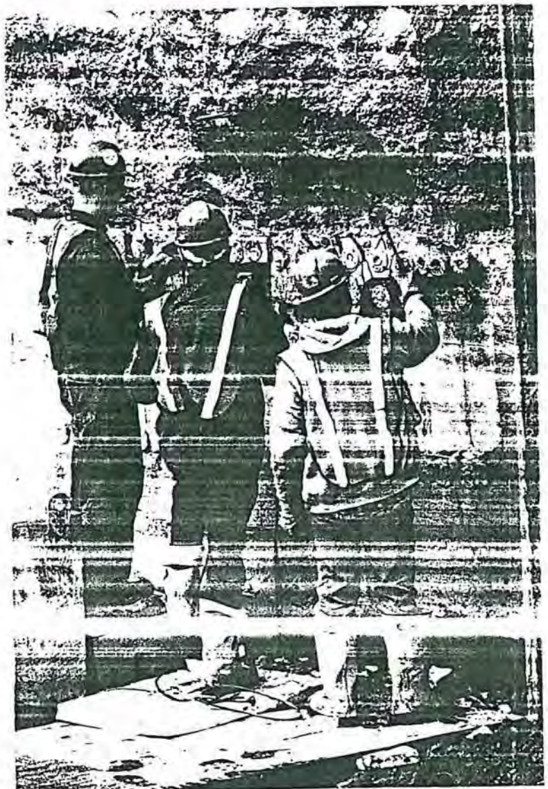
13, 14: Two views of Ironworker platform in use by Laborers removing plywood from around threaded holes in slurry wall
