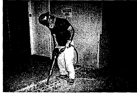
Demolition with hand-held tools
