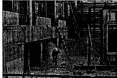
Concrete saw cutting
