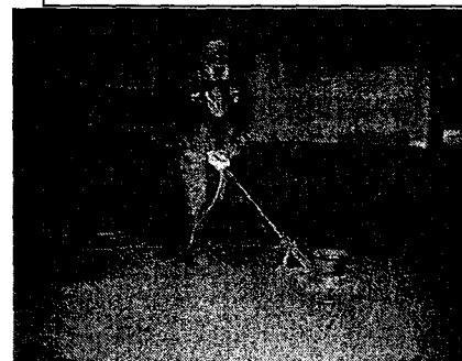
Concrete saw cutting
