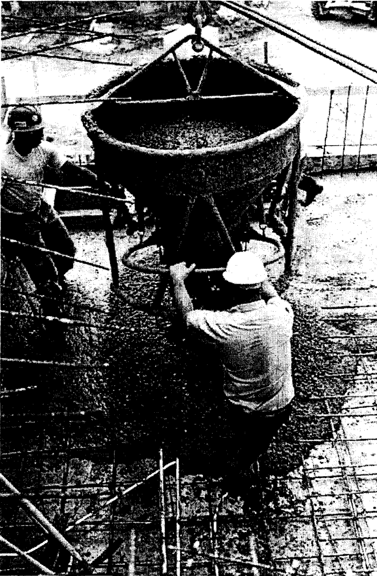
Figure 12.7 Bucket dumping operation during pouring at Beckley WV.
