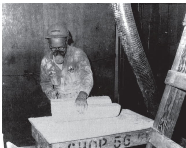
Figure 3. Work area of insulator sawing pipe insulation on a table. Photo Source: Carl Mangold. Previously published in Hollins et al., 2009.
