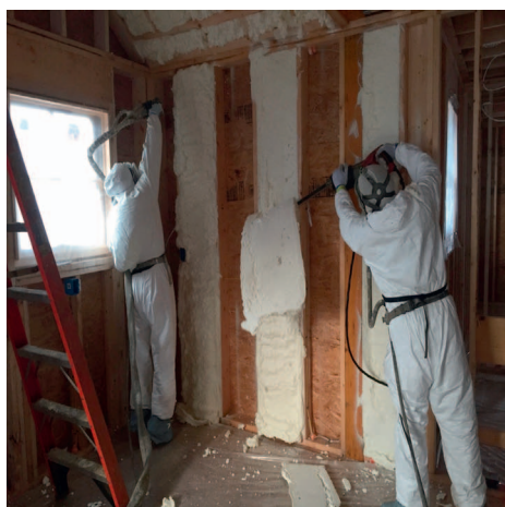
(a) Spraying and shaving of foam
