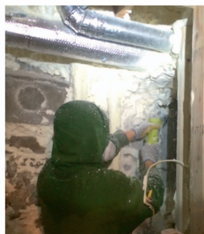
(b) Foam removal using a powered brush tool
