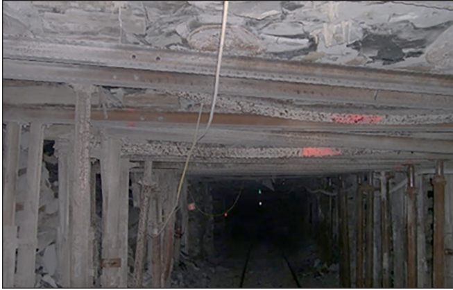
Figure 1. Steel set and posts in a track entry
