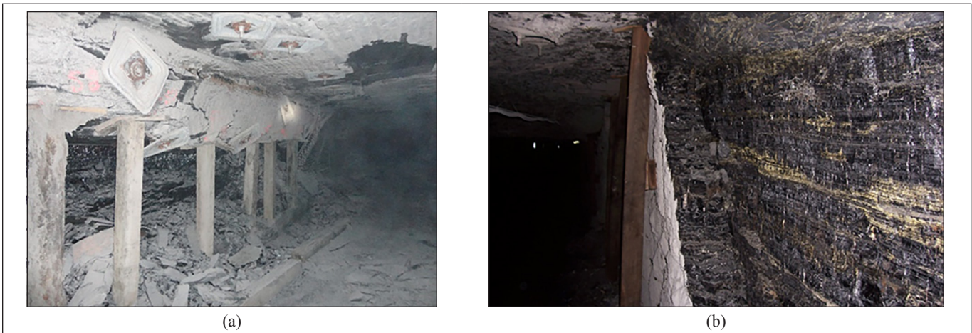
Figure 2. Standing supports used to support rib brow and to confine rib slab
