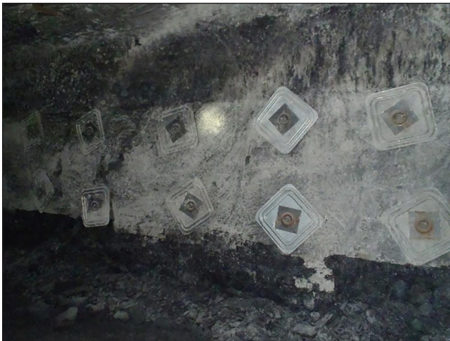
Figure 2. Photo depicting the thickness of the in-seam parting as well as showing conditions typical of the right-hand side of the study panel
