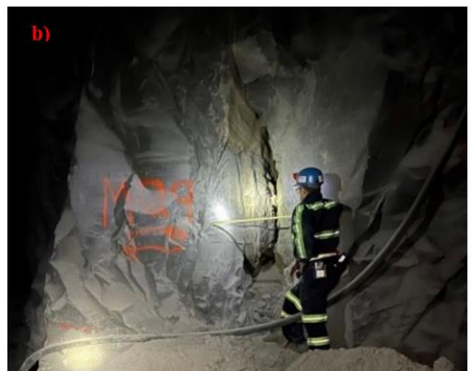
Figure 4: Karst cavities of different sizes observed nearby the collapsed area in the study mine: a) small size and b) large size.
