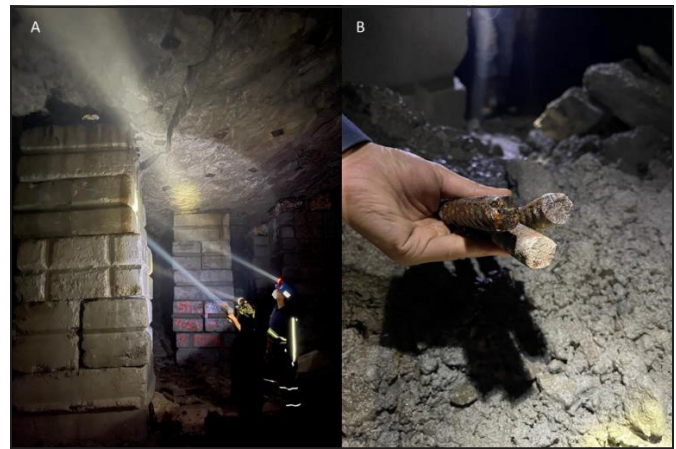
Figure 6. A) Photo of shear failure in roof and B) Photo of sheared bolts
