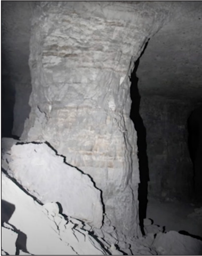
Figure 2. Hour-glass shape of pillars left after benching
