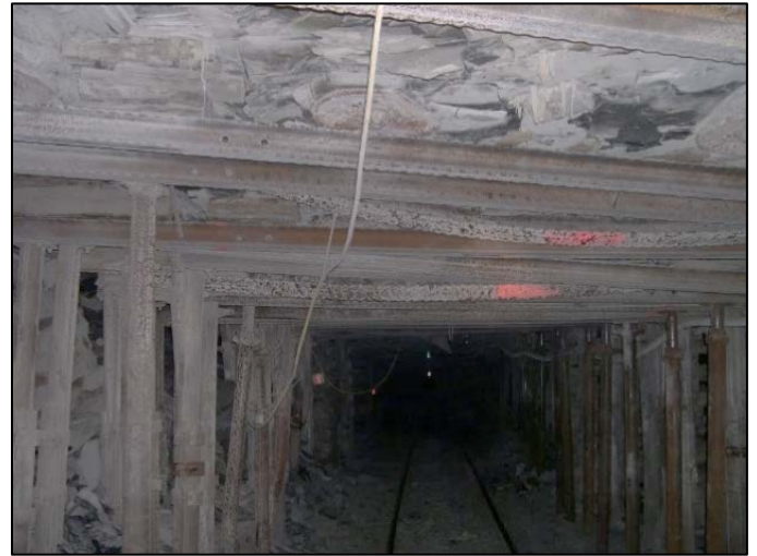
Figure 1. Steel set and posts in track entry
