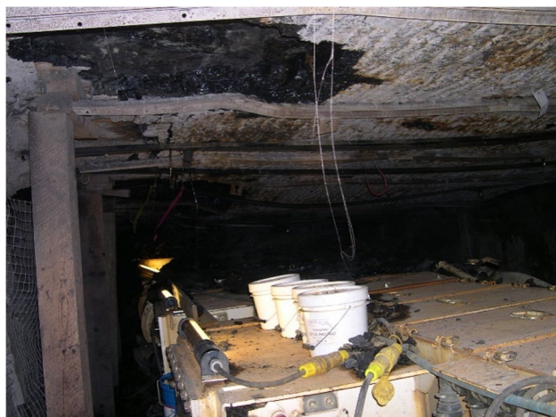
Fig. 5 Roof cutter developed at the belt entry corner on the chain pillar side
