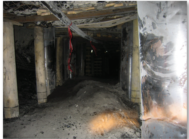
Fig. 1 Floor heave observed in the underground coal mine.
