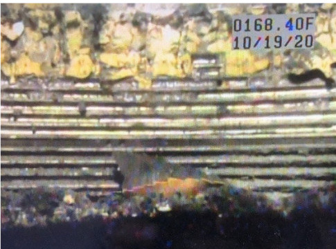
b. Lateral view of the casing wall with coupler joint exposed.
