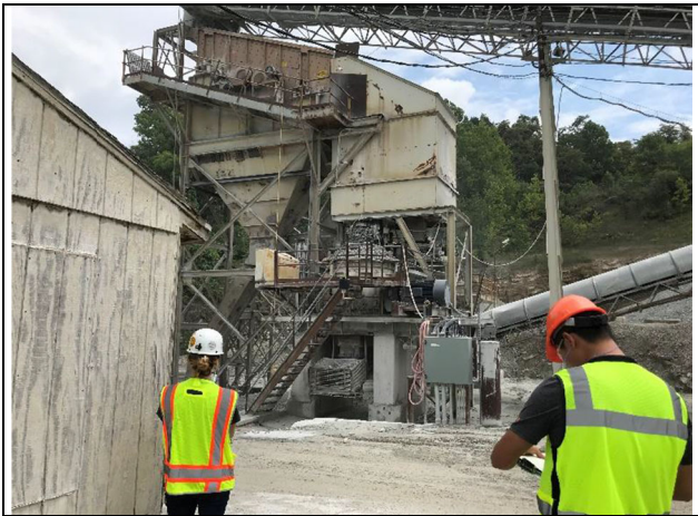
Fig. 29 Outside area in the lower processing plant near crusher/screening structure
