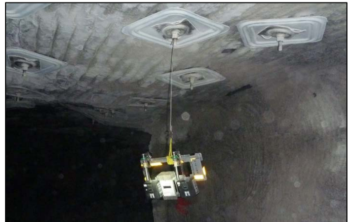
Figure 3. A typical sampling package consisting of a pDR and two gravimetric samplers. This package is typically hung from a roof bolt.
